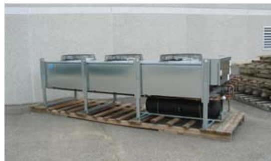
Air cooled condensers are sized by ESPEC to match the refrigeration system, but should be installed as close as possible to the chamber to ensure best performance.
